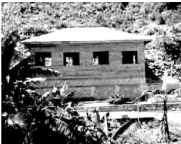
The meeting house in Mandeville under construction.
